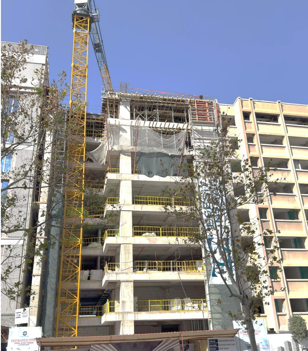
BUSINESS CENTER İNŞAATI
